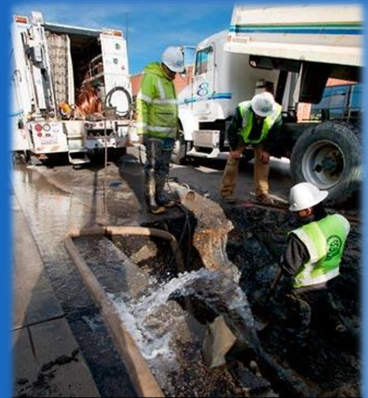
EBMUD Leak Detection
