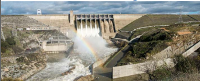
Folsom Dam project funded by Prop 18 – with five spillgates open, releasing water to the American River in Folsom, CA — December 2016
